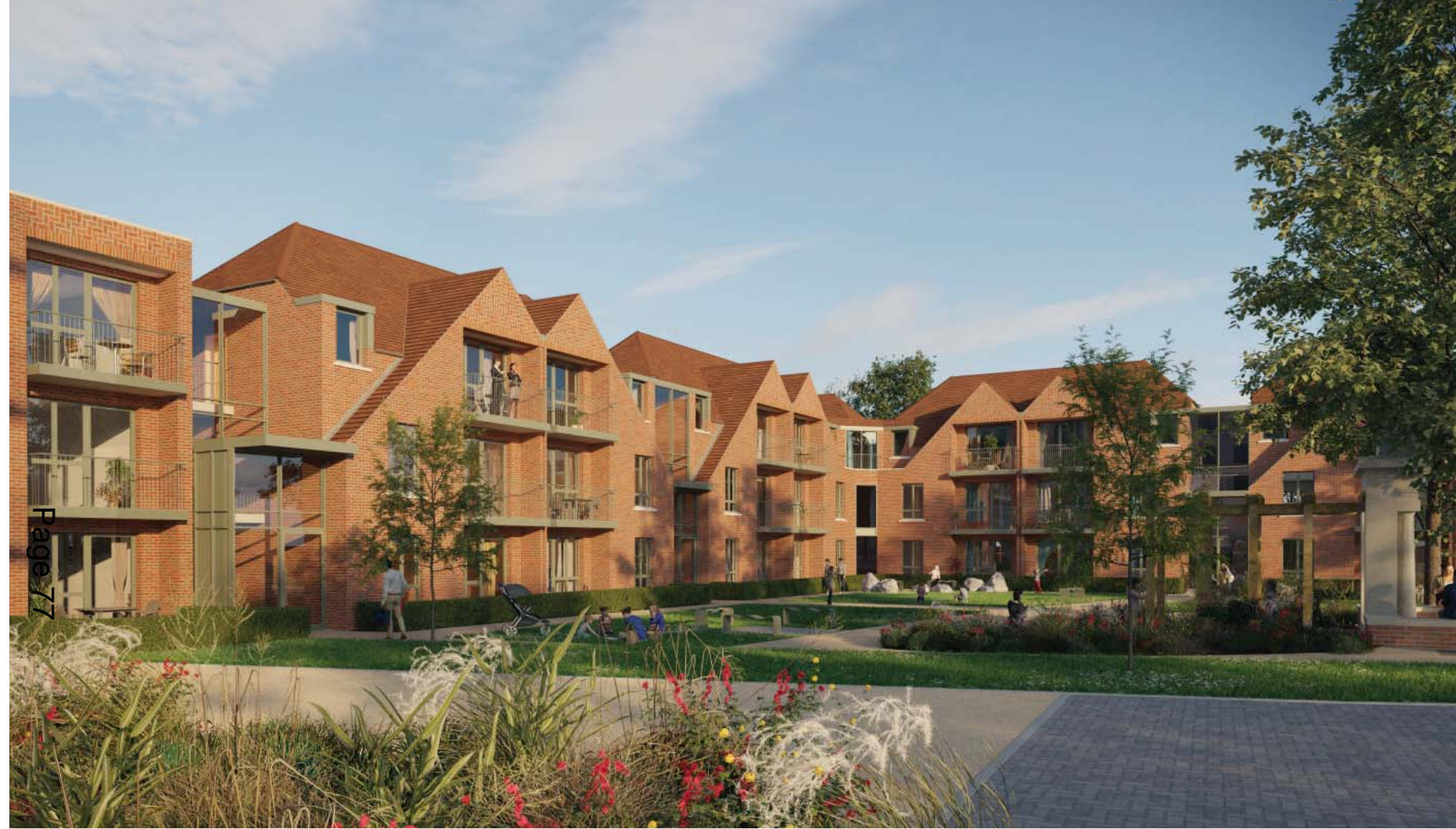
FIGURE 4.33 - VIEW TOWARDS POCKET PARK & PLOT B
